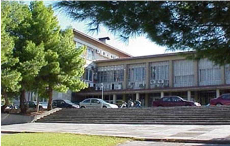
Figure 1: Building B of the Computer Engineer Department
